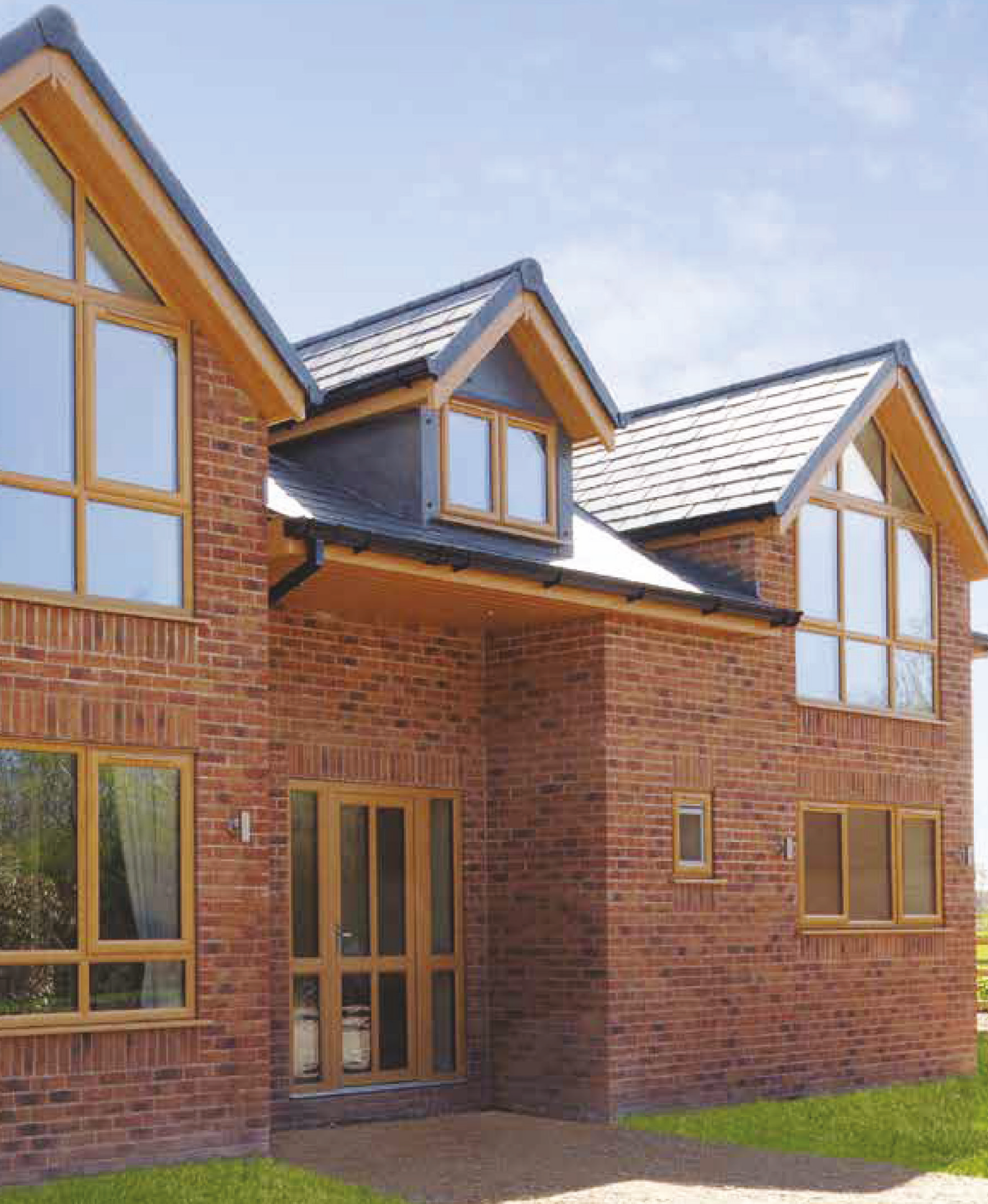
Detached property featuring square fascia and plain flat soffit boards in Irish Oak Finish, with matching windows.
