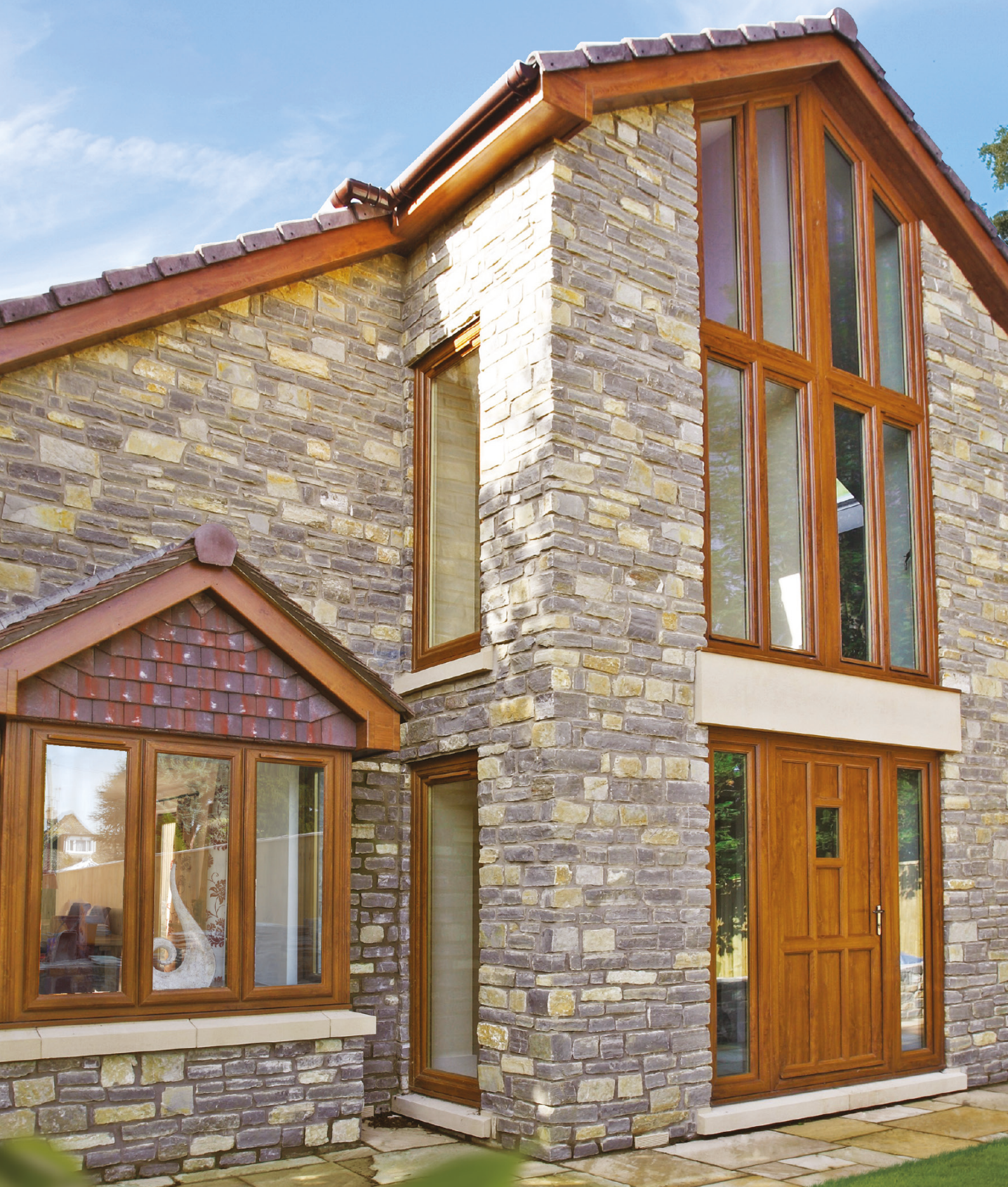
Golden Oak square fascia boards and grooved soffit boards Universal XL guttering in brown is complemented by dry verge, also in brown.
